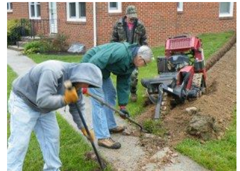
Jesse Yates, Ed Williams, and Bill Appleton working on the trench to the Food Ministry building
