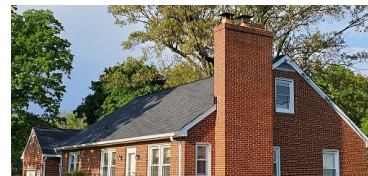
The parsonage roof was replaced on Apr. 26.
